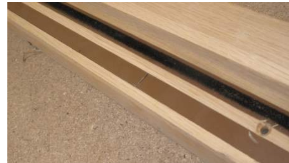
Example of replacement seal with tight butt joints.
