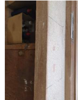
Epoxy wood filling product applied, filling gaps of up to 1mm.
