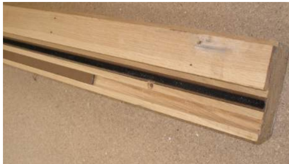
Example of damaged or missing seal.
