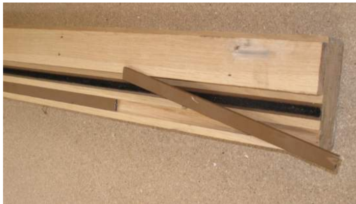
Example of seal falling away from groove
