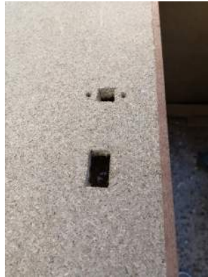
Edges of the void squared such that timber sections fully fill the area.
