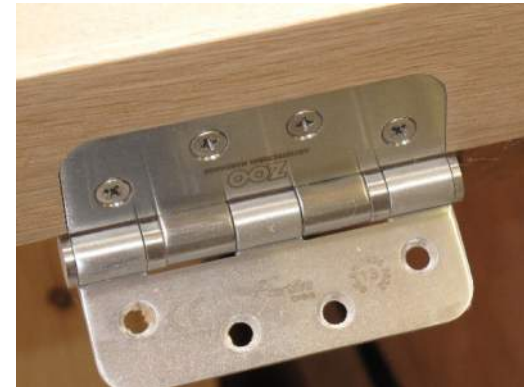
Example of an alternative hinge fitted in place of the previously removed damaged hinge.
