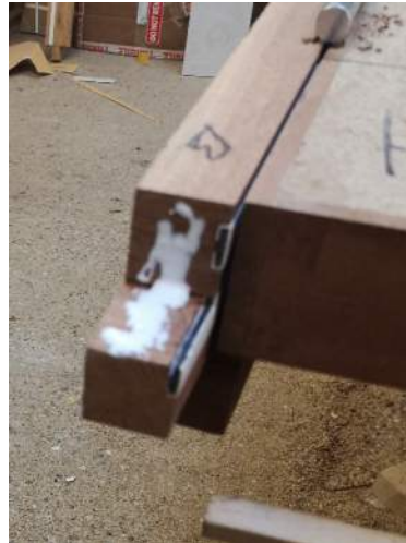
Application of PVAc (Type D3) adhesive to re-made joint within workshop conditions.
