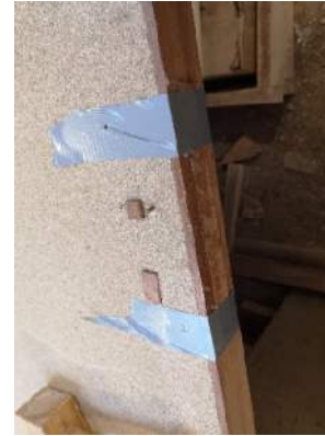
Timber sections applied to the leaf & frame.
